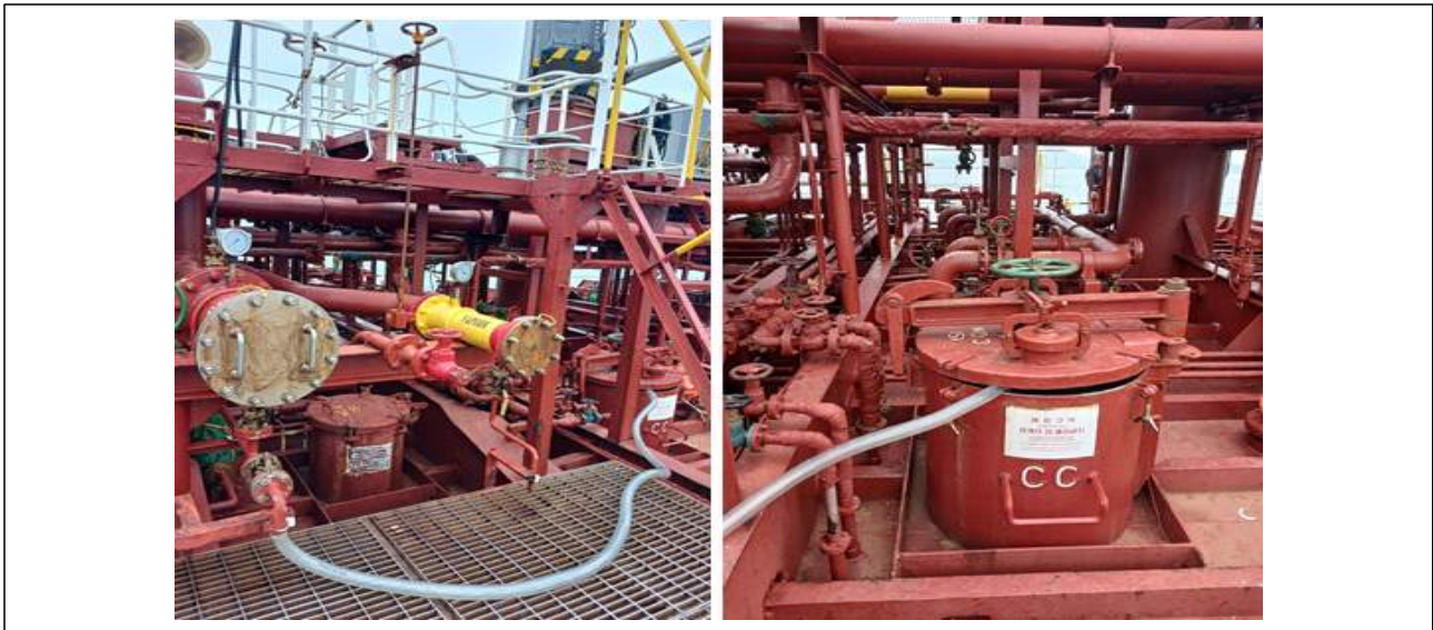
<Figure 9> Recreating the operation of connecting hoses for air blowing on board New Global (which belongs to Seongho Shipping; and the photos were quoted from the company's documents)
