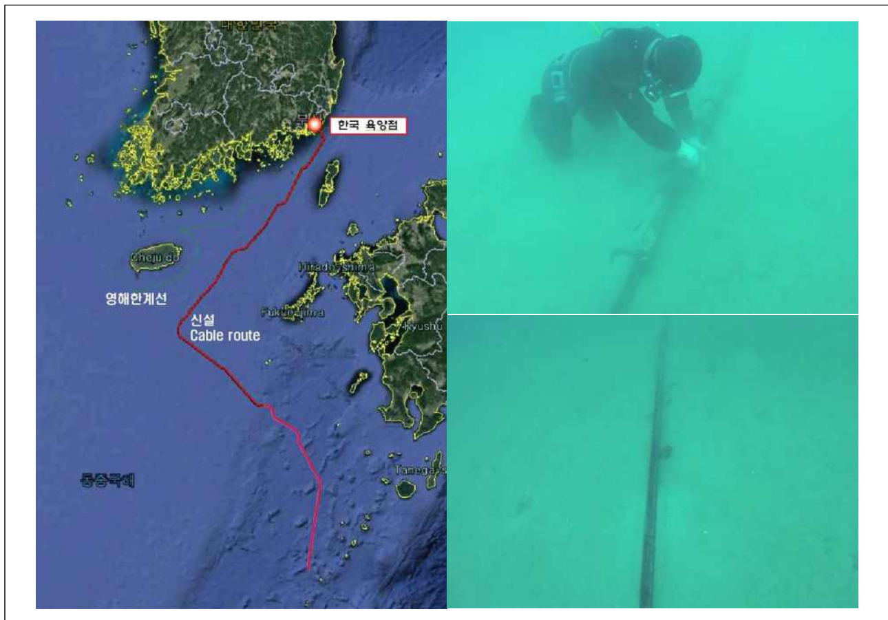
<Figure 14> Cable laying route and photo of construction
